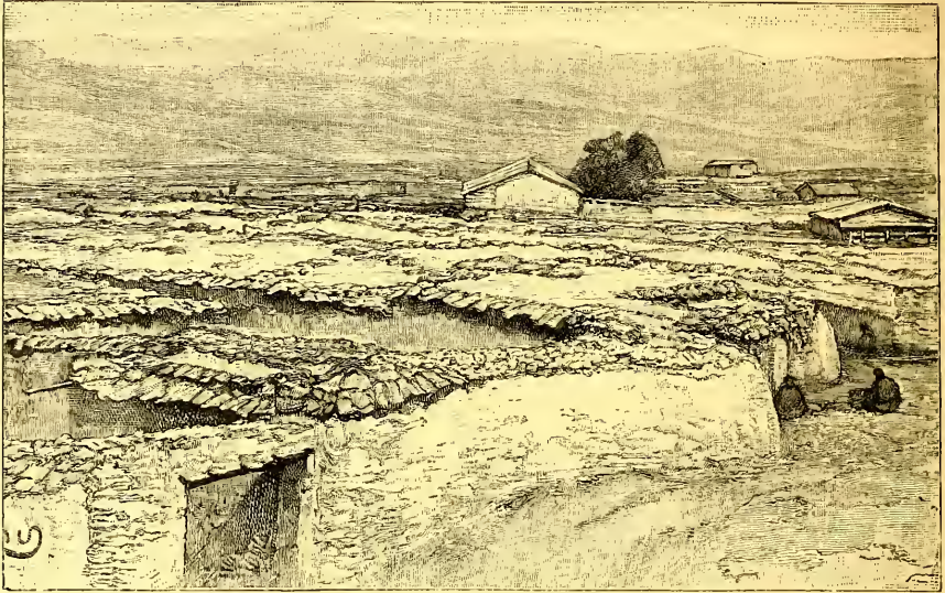
LITANG: VIEW FROM THE ROOFS.
